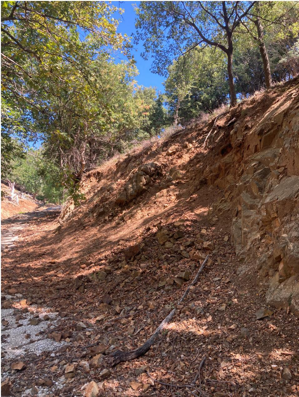
Figure 1: Collapsed soil slipping onto a cement road, Samothraki, August 2022.
